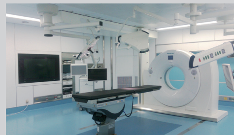
The P1-55 unit is fully embedded into one wall of the operating room and equipped with a built-in 55" monitor featuring a high-brightness display at a full HD 1920 x 1080.
